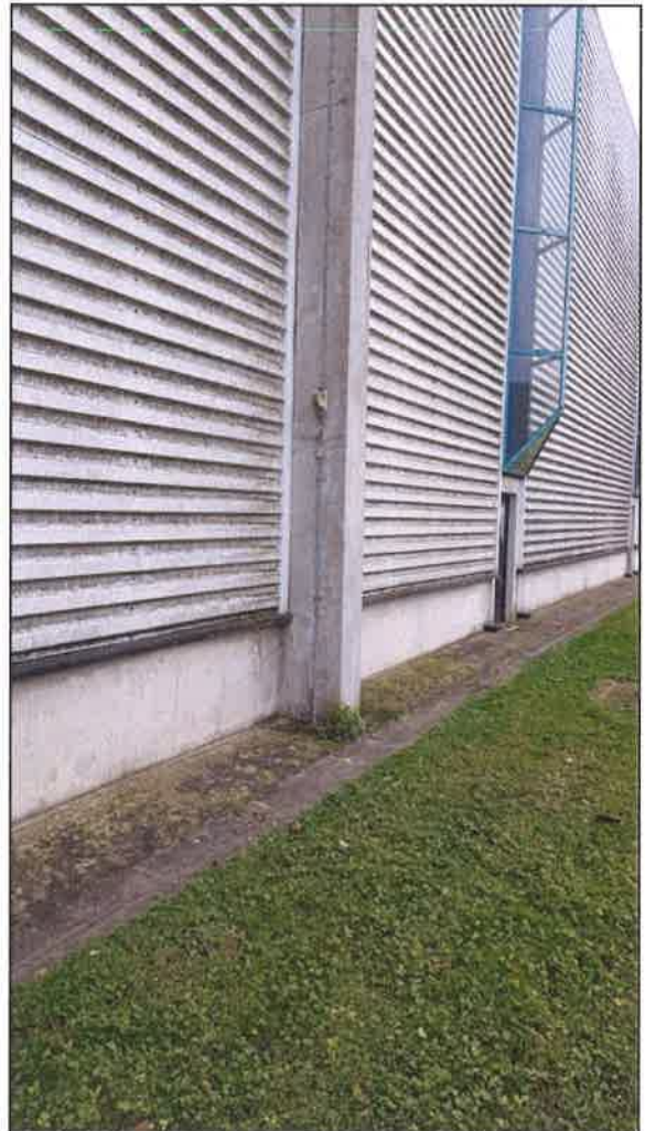
Installation PDA n°5
