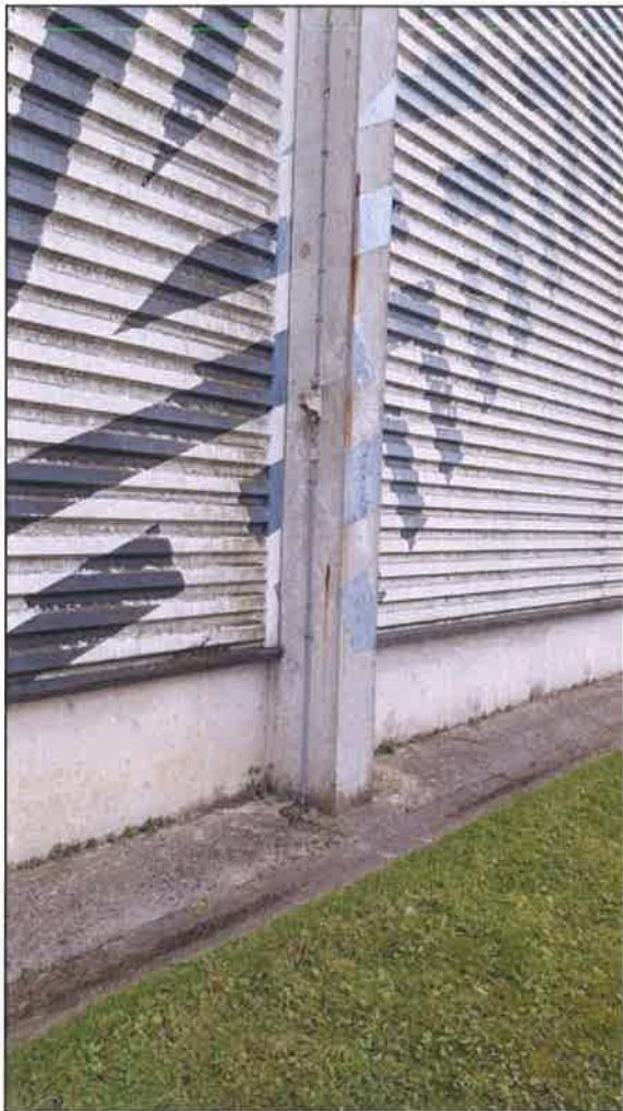
Installation PDA n°4
